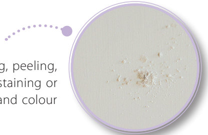
Any blistering or mould growth on painting
