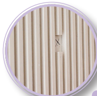
Missing door viewer
