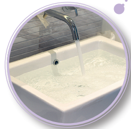
Simple flooding test for sink and wash basin to verify the effectiveness of overflow pipe and joint sealant
