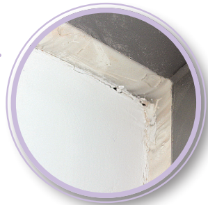
Any signs of chemical or cement remains, oxide residue, discolouration on window frames
