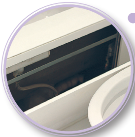
Examine the condition of maintenance chamber under bathtub
