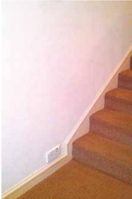
Picture 8a Switch at Low Level
