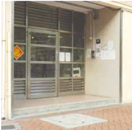
Picture 6a No Ramp at Entrance
