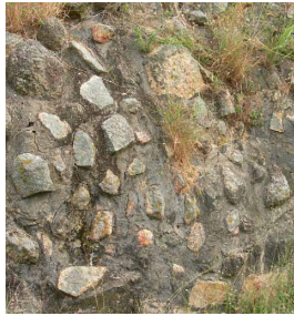
Rubble stone wall
