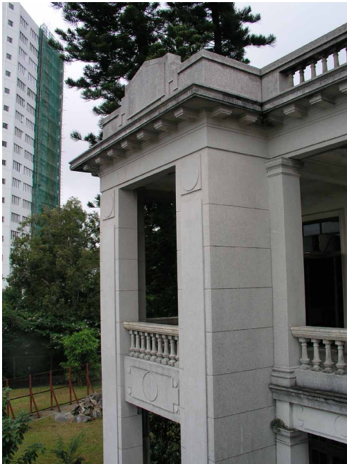
The Shanghai plaster wall finish
