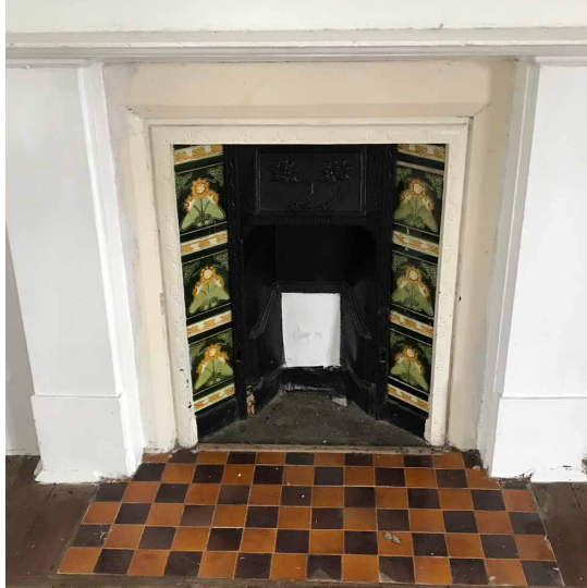
The incorporation of glazed ceramic tiles in fireplace
