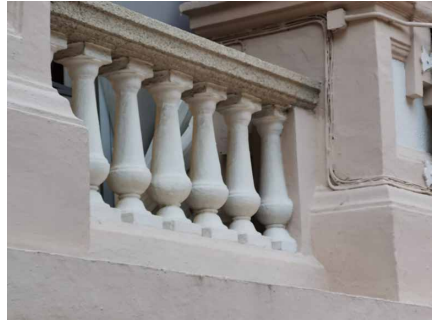
The baluster of the Main Building, the University of Hong Kong.
