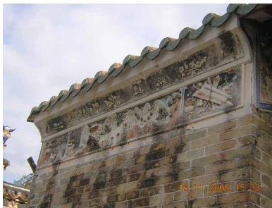
Running water stains can be reduced if water drip lines or grooves are formed at the upper frame of the plaster decoration.
