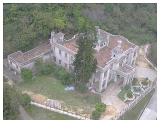
Jessville at Po Fu Lum Flat roof of Western residential house covered with canton tiles
