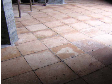
Terra cotta Canton tiles paving in a side chamber of a Chinese house
