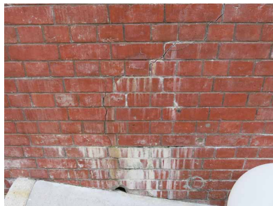
Running water stains can be reduced if water drip lines or grooves are formed at the upper frame of the plaster decoration.
