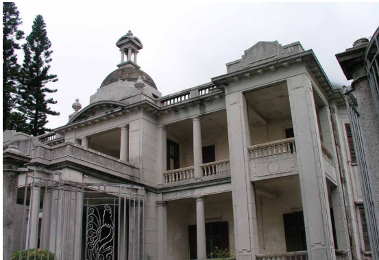
Towers on the roof of Jessville
