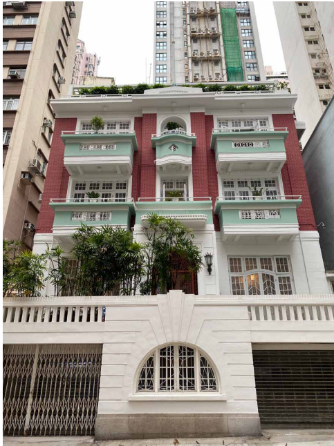
Modern paint used on tong lau
