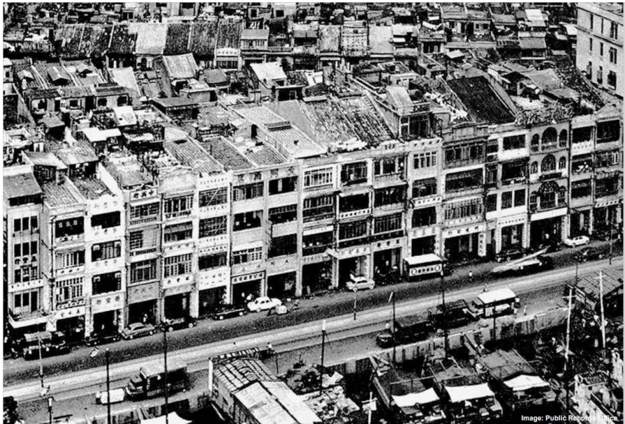
Photo of Sheung Wan in early 20th century showing different-generations of Tong Lau. The top part of the photo shows large groups of Tong Lau without back lanes.
