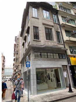
No. 51-53 Yen Chow Street, Sham Shui Po (left) The grade 3 historic tong lau was built in 1933 and it is currently an art exhibition venue. It is at 4 Second Lane, Tai Hang. (right)
