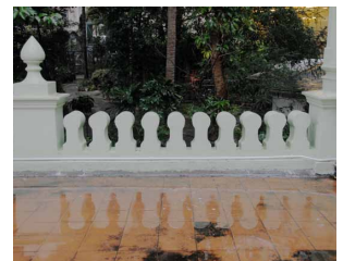
Flooding at roof due to blocked drain and downpipe
