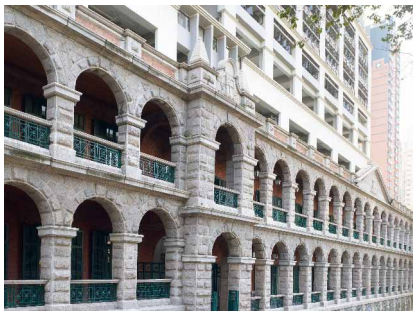
Stone facade of Old Mental Hospital (1892)
