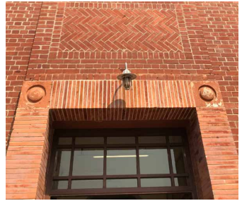
Red brick wall
