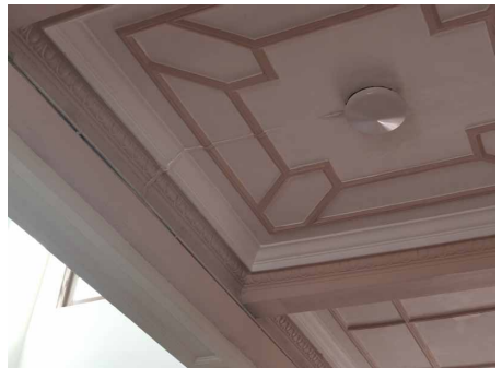
Distemper ceiling of the Main Building, the University of Hong Kong.
