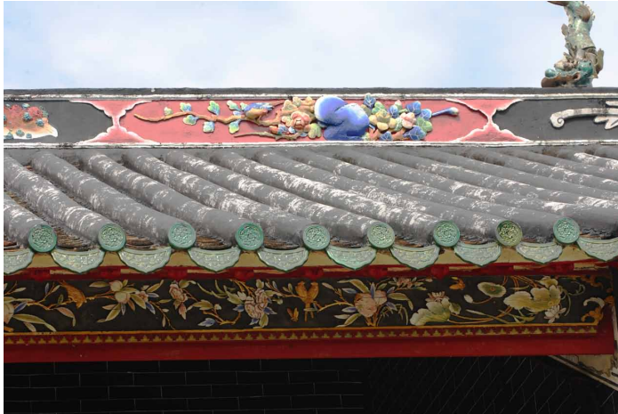
Cap tiles and drip tiles at the eave of the roof
