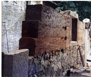
Rammed earth wall
