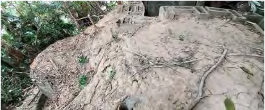
Figure 9: Roof of the structure showing two ventilation shafts made of drainage pipes and part of the possible LAAMG post (10 February 2022 by Lawrence W. C. Lai)
