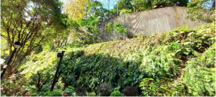
Figure 2: The retaining wall (8 February 2022 by Lawrence W.C. Lai)
