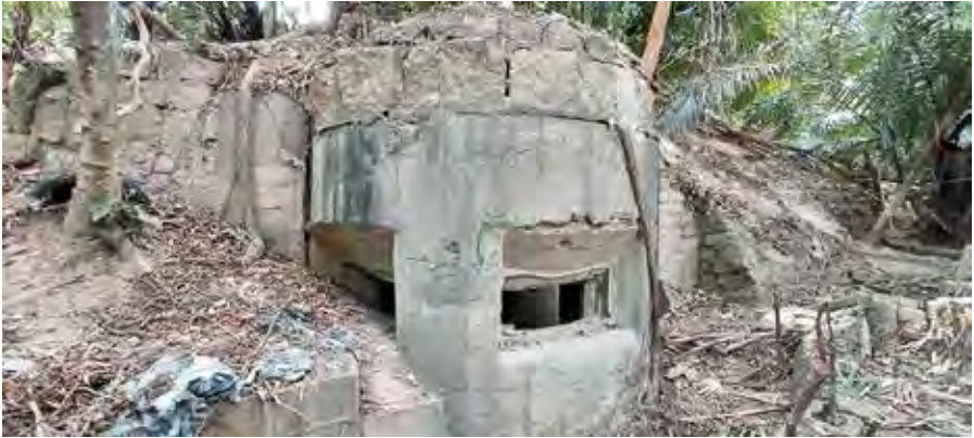
Figure 4: A side view of the front of the structure showing two of its embrasures, its granite block-capping and the stone revetments of the rear chamber (8 February 2022 by Lawrence W. C. Lai)
