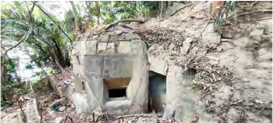
Figure 5: A side view of the front of the structure showing its entry (8 February 2022 by Lawrence W. C. Lai)
