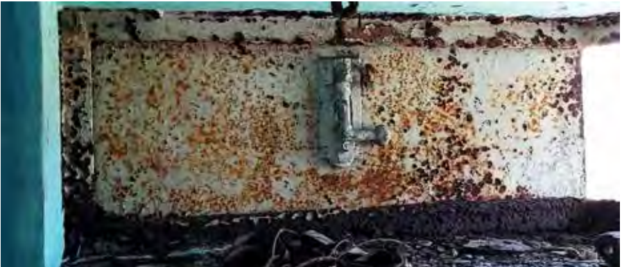
Figure 31: The locking mechanism of an aperture shutter of OP Middle Gap (1 November 2021 by Lawrence W.C. Lai)
