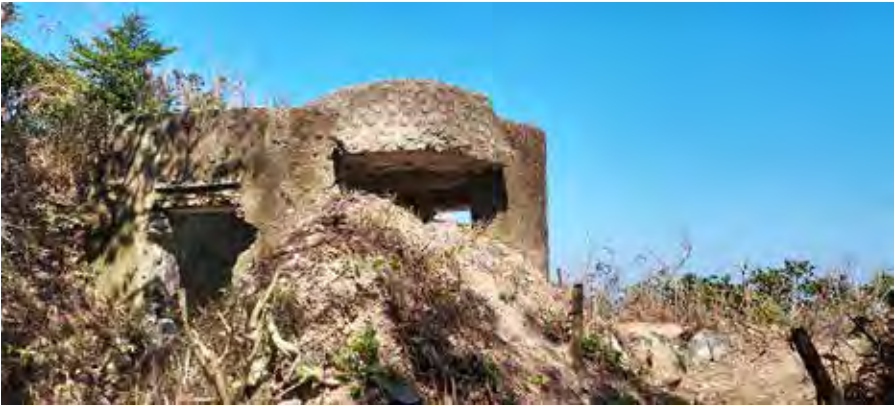
Figure 7: Side view of Pottinger Peak OP showing the entrance (6 February 2021 by Lawrence W.C. Lai)
