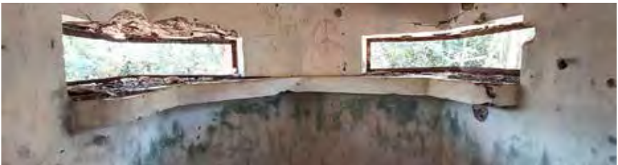
Figure 58: Interior view of OP Middle Spur
