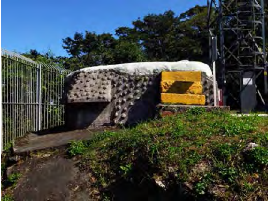
Figure 35: Exterior left side view of OP Victoria Peak (29 November 2021 by Lawrence W.C. Lai)
