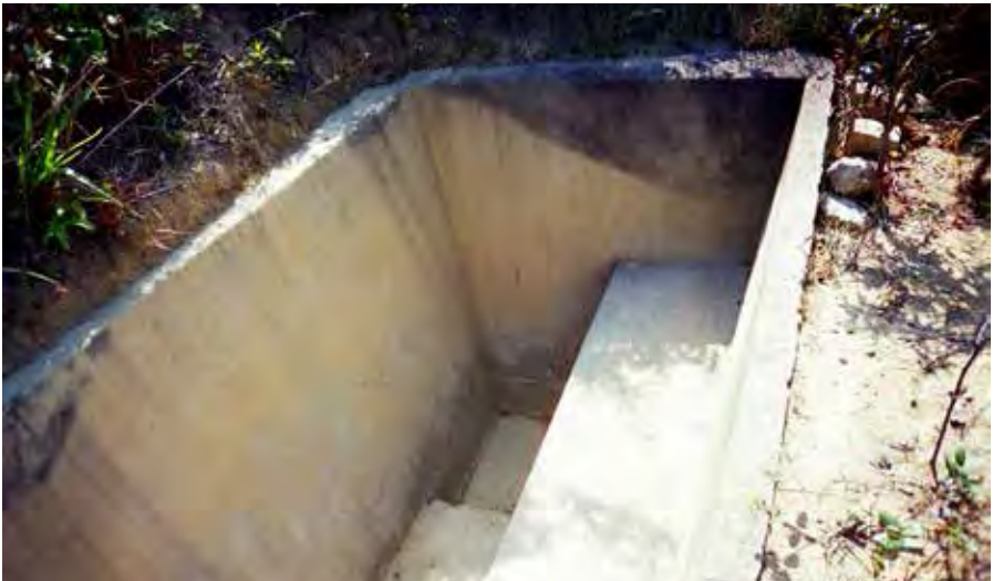
Figure 11: Fire trench (T3), its southern end (Taken by the second author on 26 December 2007)
