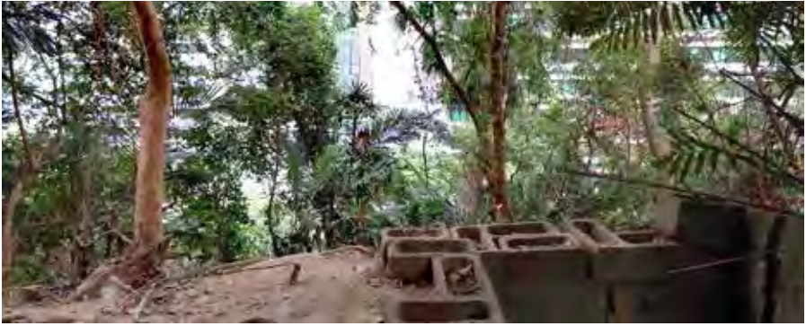
Figure 8: View of the Harbour from the roof of the structure with a rectangular, low-walled, open-backed location (possibly a LAAMG post) on the right (10 February 2022 by Lawrence W. C. Lai)
