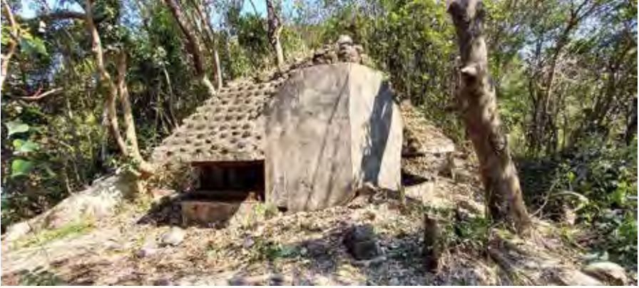
Figure 54: Exterior front view of OP Middle Spur (17 February 2021 by Lawrence W.C. Lai)
