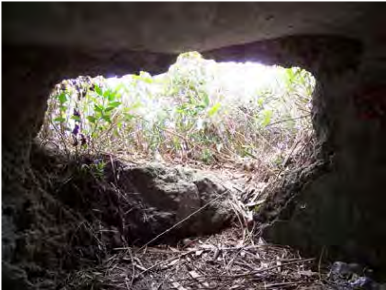
Figure 22: Damaged aperture of OP Jardine's Lookout (13 February 2008 by Lawrence W.C. Lai)
