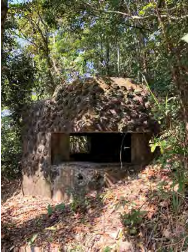
Figure 48: Left side view of OP Matilda (1 February 2021 by Lawrence W.C. Lai)
