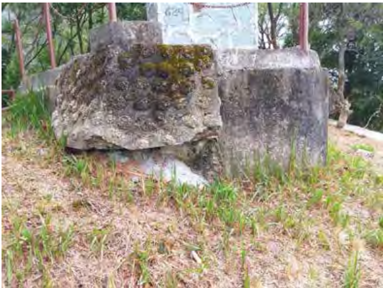
Figure 41: Exterior right front view of OP High West (31 December 2021 by Lawrence W.C. Lai)
