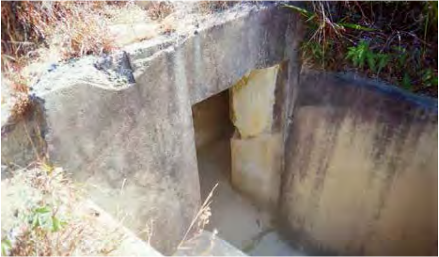
Figure 10: Fire trench (T3), part immediately outside the Kitchen of SMR (Taken by the second author on 26 December 2007)
