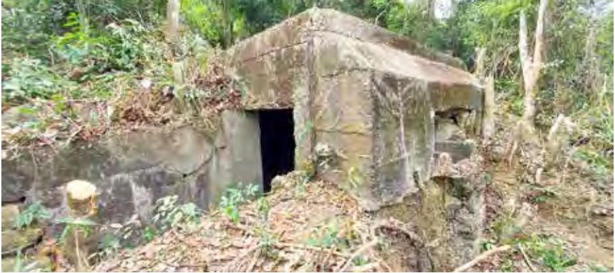
Figure 7: Right side view of OP Shaukeiwan (Shau Ki Wan) showing its entrance and the protruding lower part of the observation aperture (31 December 2021 by Lawrence W.C. Lai)
