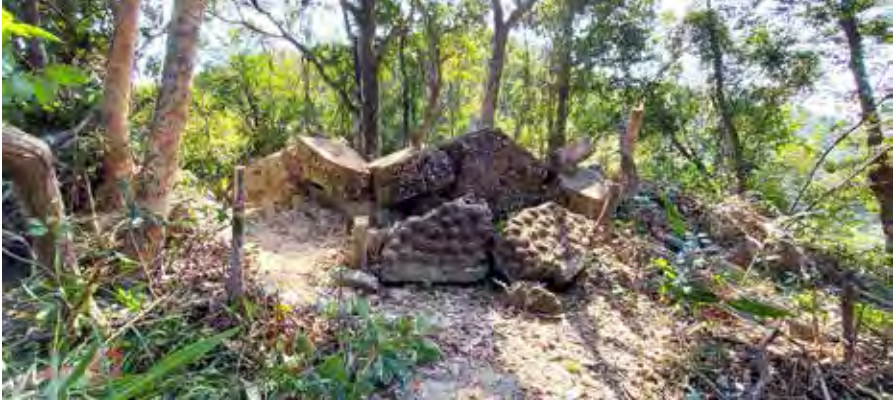
Figure 33: Exterior front view of OP Wanchai Gap (3 February 2021 by Lawrence W.C. Lai)
