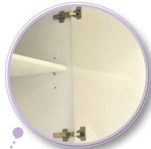
Any missing or loosen hardware such as handles, hinges, magnetic catches and supports
