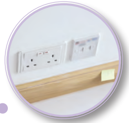
Examine the electricity supply to lighting fittings and plug-in sockets
