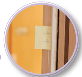
Loosen joint at door frame
