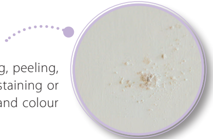
Any blistering or mould growth on painting
