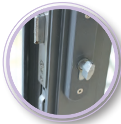
Any signs of missing, deformation, loosen ironmongeries such as window fastener
